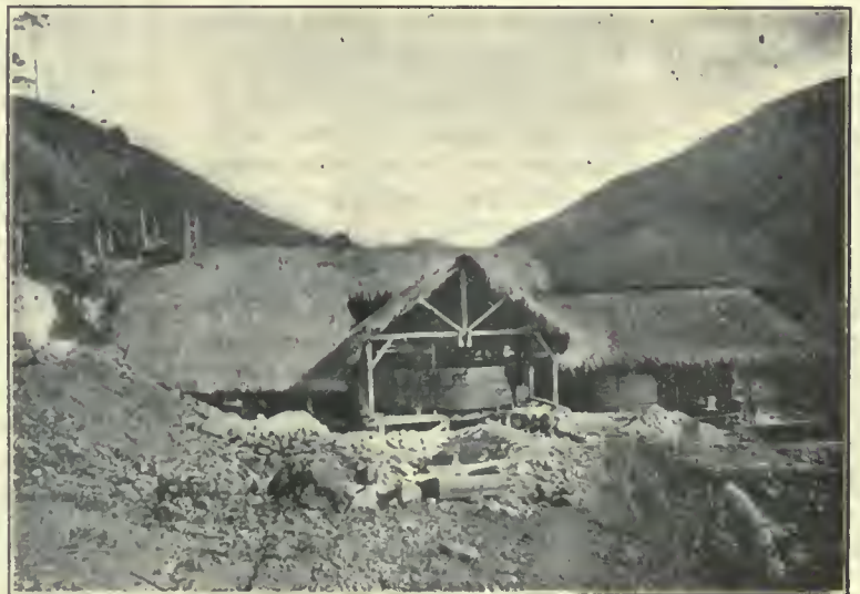
BENGUET CONSOLIDATED MILL. GRASS ROOF LATER REPLACED BY IRON.
